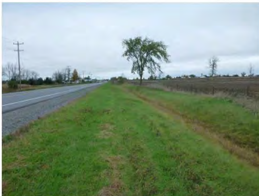
Image 13: Ditched right-of-way of County Road 31, view northwest.
