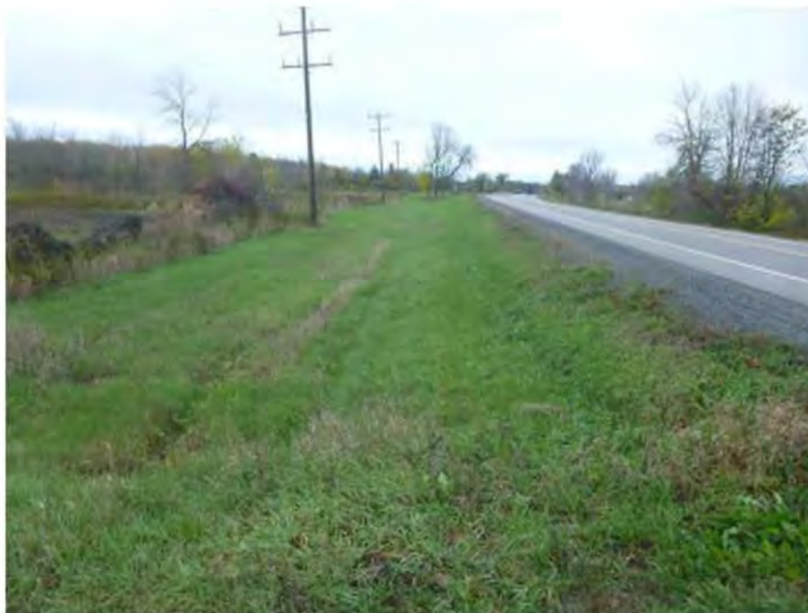
Image 22: Right-of-way of County Road 31, view southeast.
