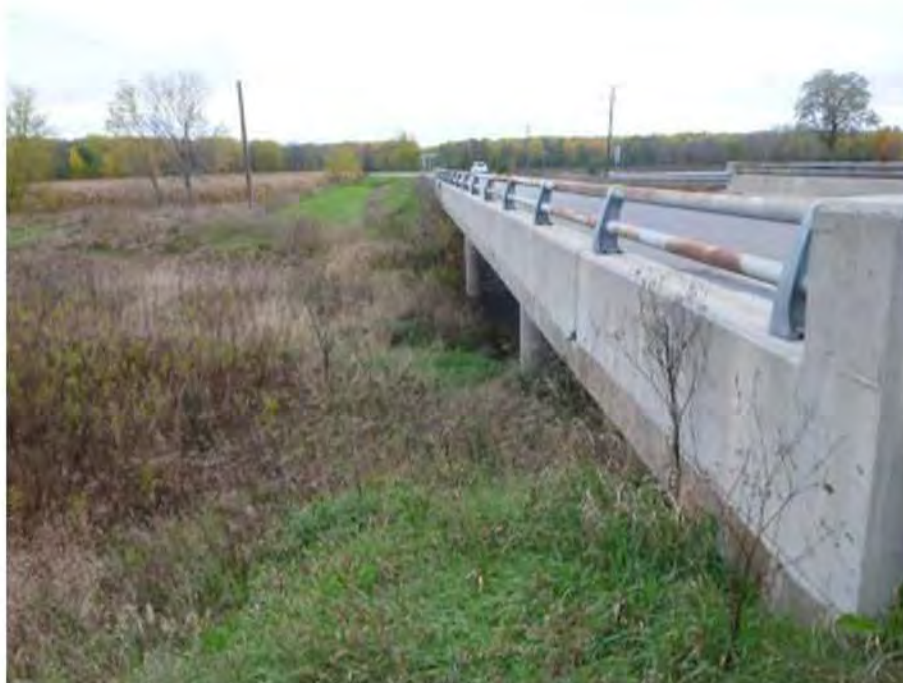
Image 19: Bridge over McMartin Drain, view northwest.
