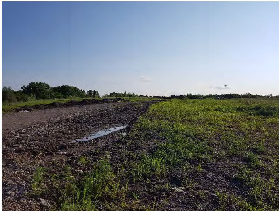
Image 3: View southwest showing conditions within the Boyne Road Landfill.
